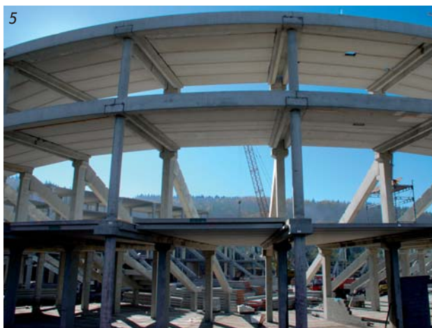
Fig. 6 Placement of bended spandrel beams – general view
