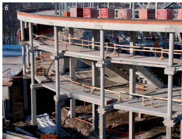
Fig. 6 Placement of bended spandrel beams – general view
