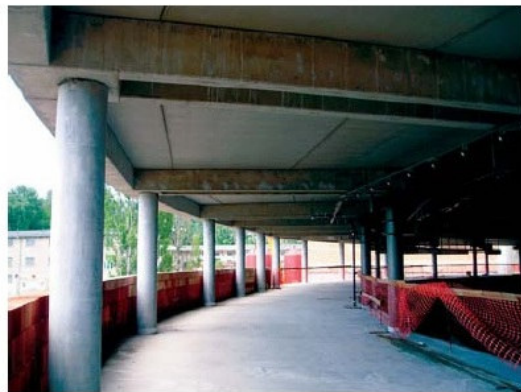
Fig. 8 Tectonic of floor structure in the rounded part
