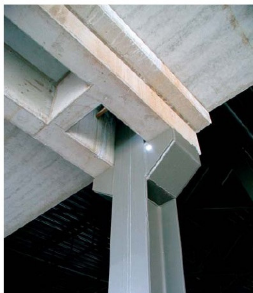
Fig. 6 Twin beam with an opening for wiring and piping placed on a steel column carrying the roof cover of the hall
