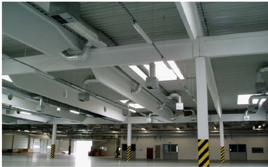
Fig. 8 Piping in the hall with a grid of 12/24 m Obr. 8 Technická rozvody v hale s rozsedem 12/24 m
