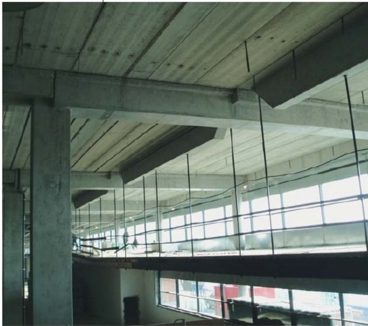
Fig. 7 Arrival corridor with steel gallery hung to the prefabricated floor structure
